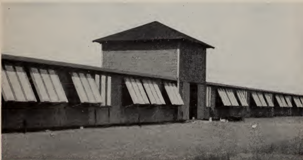
Fig. 13. Three-purpose curtain, showing some curtains closed down, and some extended at bottom for ventilation. Fig. 63 shows this same type of curtain with inner panels open to admit sunlight.
